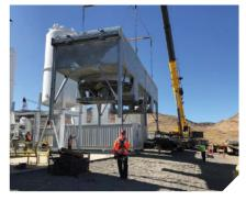
As well as the delivery, C.H. Robinson's onsite logistics representative also oversaw many other aspects of the project, including shrink wrap removal, purging gas from vessels, shifting bollards to widen the approach, security staff communication and shuttling drivers to evaluate entry options.
