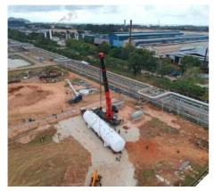
another team of Megalift's was stationed in Petronas's chemical plant to perform the ground preparation work including removal of fences and laying down of steel ramps and plates. On arrival, the 82th pressure vessel was then lifted and placed onto its foundation using a 500th crane – all handled by the expert Megalift heavy lifting team.
