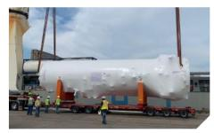
H. Robinson Project Logistics helped transport 2,000cbm of LNG equipment from China to Texas for a chemical plant expansion. The project involved a part charter and approximately 65 domestic truck loads, including breakbulk pieces, containers, crates and loose items. The largest piece was a H2 liquefier cold box which weighed 86.82mtn and measured 18.52 x 4.70 x 4.85m.
