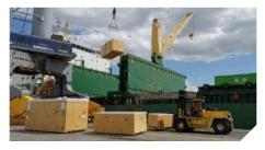
C.H. Robinson Project Logistics recently undertook a door-to-door project for a long-time valued customer. A total of 800cbm of crated liquid natural gas (LNG) equipment needed to be moved from a supplier in Poland to the site in Mexico. The largest piece on this heavy lift move was a refrigeration unit, which measured  $7.35 \times 2.65 \times 5.31$ m and weighed 20.3mtn.
