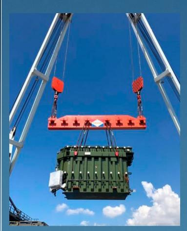
The transformer weighed 167tn with dimensions of 830 x 330 x 450cm. NTG handled the whole job including, not only transporting the main transformer, but also hiring specialised gear and manpower for the installation work at the site, along with moving urgently needed anti-vibration pads on a dedicated truck from Italy to ensure the timely installation in Denmark.
